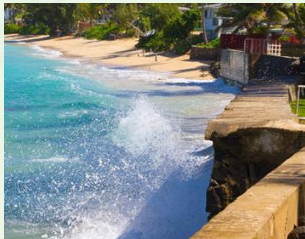
Figure 2 - Shoreline armoring in Hawaii have resulted in beach loss, bringing forth a "no tolerance" policy towards new seawalls. Photo Credit: Grist/joshuaraineyphotography / Getty Images
