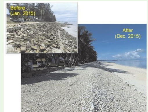
Figure 22 – Tuvalu's government strategically dredged and placed gravel and sand on Fongafale Island.
