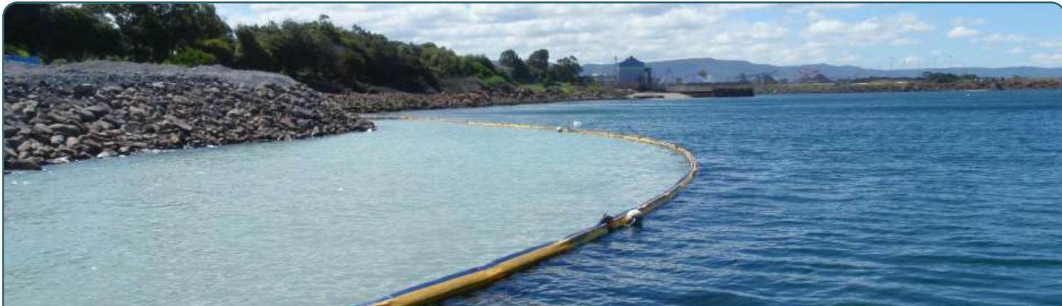
A silt curtain contains the soils and sediments disturbed during coastal construction.
