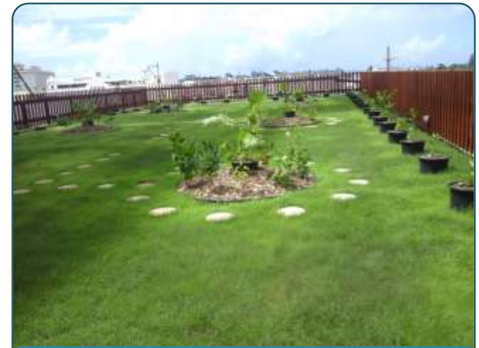
THIS: A green roof on Saipan helps reduce stormwater runoff and has added benefits of lowering energy costs and reducing humidity in the building.
