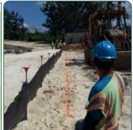
THIS: Anchor and maintain silt curtain to retain dirt and sand on site.
