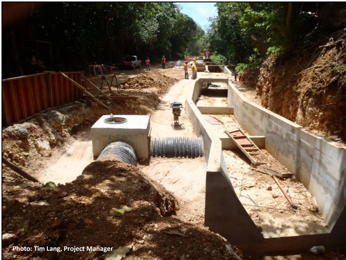
FIGURE 6: LaoLao Bay Rd. Catchment Basin System with Terminal Sediment Chamber
