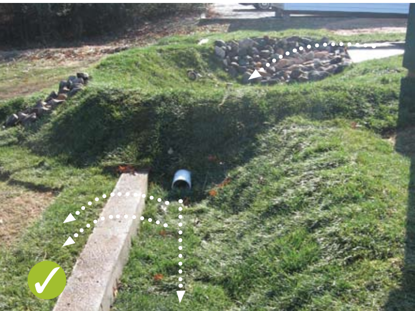
Concentrated flows are collected in small forebay and discharged into 6 inch deep "swale" before overflowing concrete lip as sheet flow (Source: NC State University).
