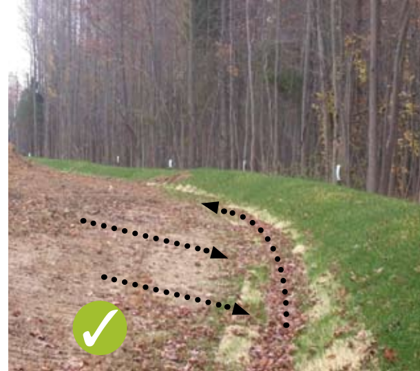
Good use of a diversion berm at the base of a slope and along the perimeter to protect adjacent natural areas from construction site runoff. The berm was stabilized with erosion control matting and grass seed.
