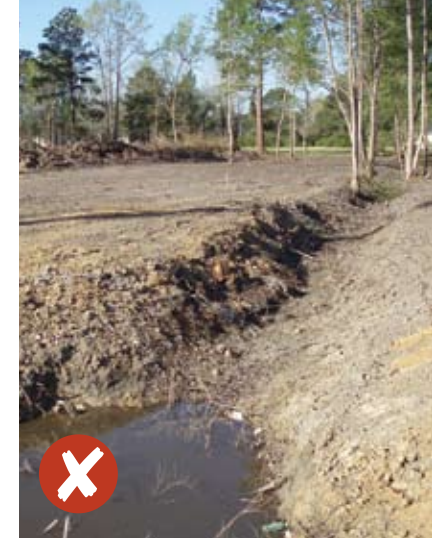
This diversion swale directs flows to a sediment trap. The slopes and surrounding area should be stabilized. Do not use swales to divert streams.
