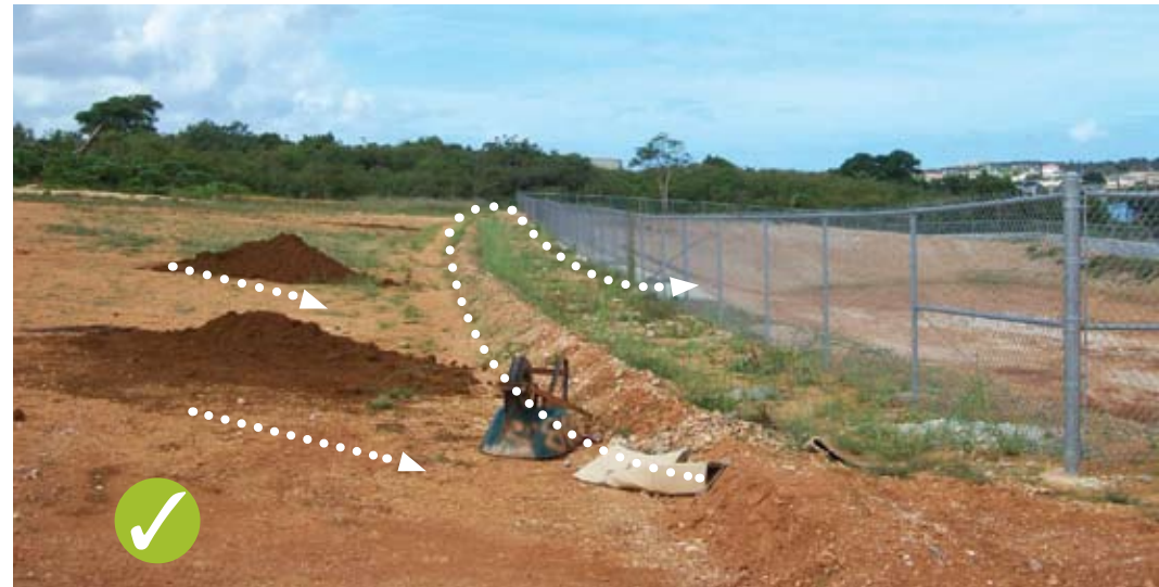
Great use of an earth berm to collect and divert runoff from the site into a stabilized outlet at the top of a ponding basin (behind chain fence on right). The berm should be stabilized with erosion control blankets or vegetation.
