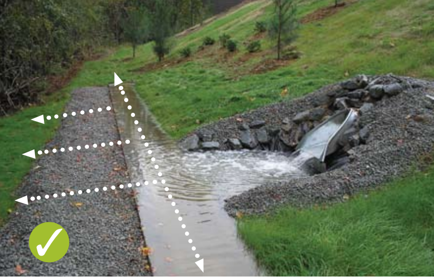
Good application of level spreader at outfall from large ponding basin. Flows plunge into small pool, spread out evenly across level concrete lip, then sheet flow from lip across gravel into grass (Source: NC State University).
