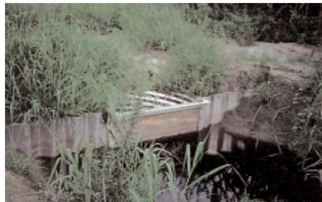
This type of flow condition commonly occurs in drop spillway structures and drop inlets with stoplogs. Refer to table 13-8.
