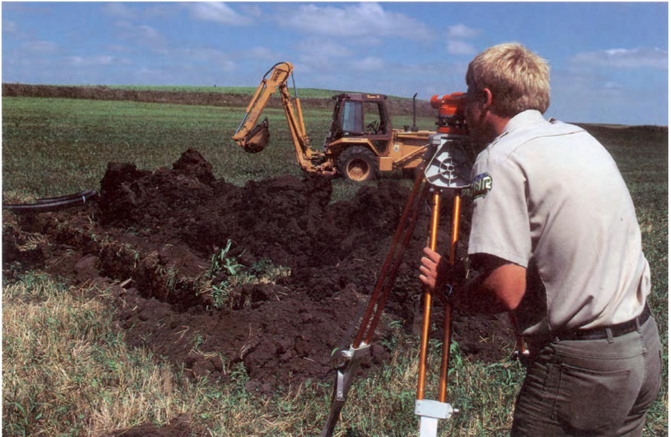
Survey data for evaluation depends upon site characteristics such as steepness of slopes, size of drainage areas, and size of the impoundment. It is recommended that enough information be obtained to plot a contour map showing intervals of 1 foot or less.
