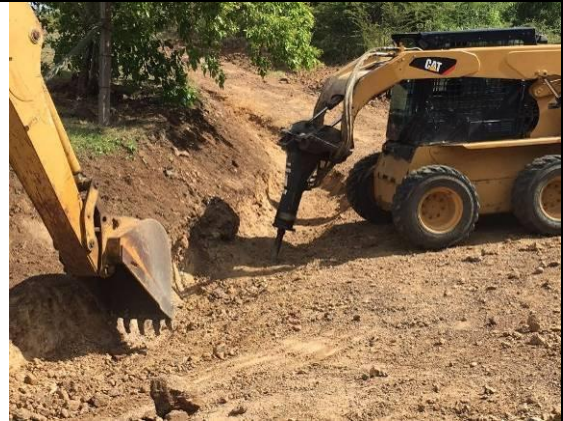
Bedrock can make ditch excavation challenging.
