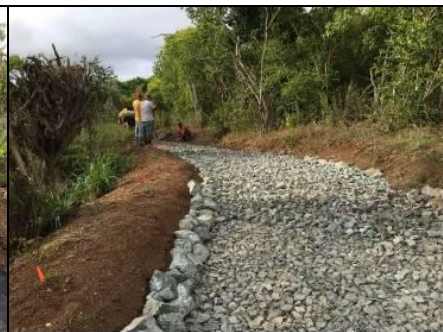
Step 3. Covering geotextile with base course.
