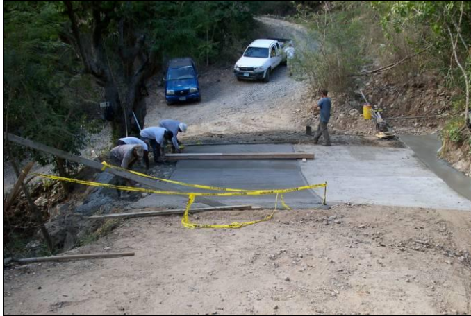
Construction of concrete dip in two pours to allow vehicular access during construction.
