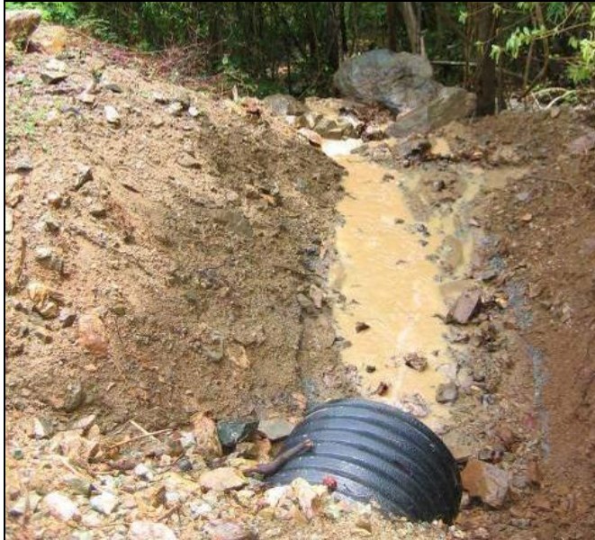
Lack of outlet protection at this newly installed cross-drain leads to erosion of slope at pipe exit.
