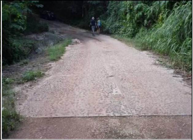
Stones embedded in concrete low-water crossing to improve vehicle traction during wet weather.
