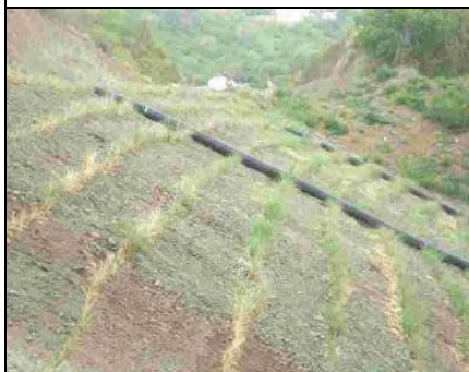
Rows of vetiver grass recently planted along road outslope. Hydroseeding is visible between rows to help hold exposed soil in place while vetiver establishes.
