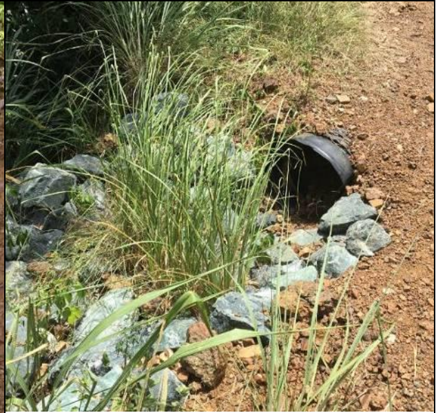
This cross-drain outlet has a stone plunge pool with vetiver grass incorporated into the berm.
