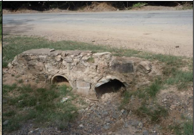
Use headwalls and endwalls (with or without wings) to protect pipe edges from damage and banks from erosion.
