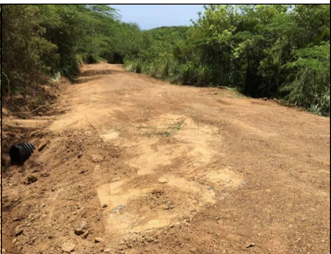
Consider adding compacted fill on top to provide sufficient cover. This could become a grade break.
