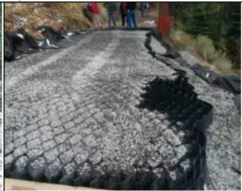
Geocells used to confine gravel at a wet area crossing on Forest Service roadway.
