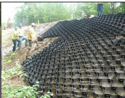
Example of geosynthetic soil containment cells used on road outslope to hold soil in place for subsequent planting.
