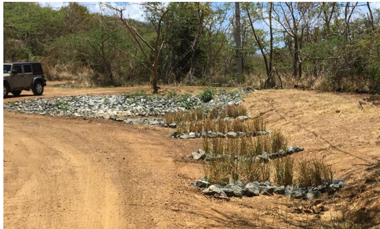
Example of recently planted vetiver-rock check dams leading to a sediment trap on Culebra, Puerto Rico.
