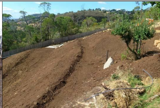
Large scale terracing prior to vegetative planting.
