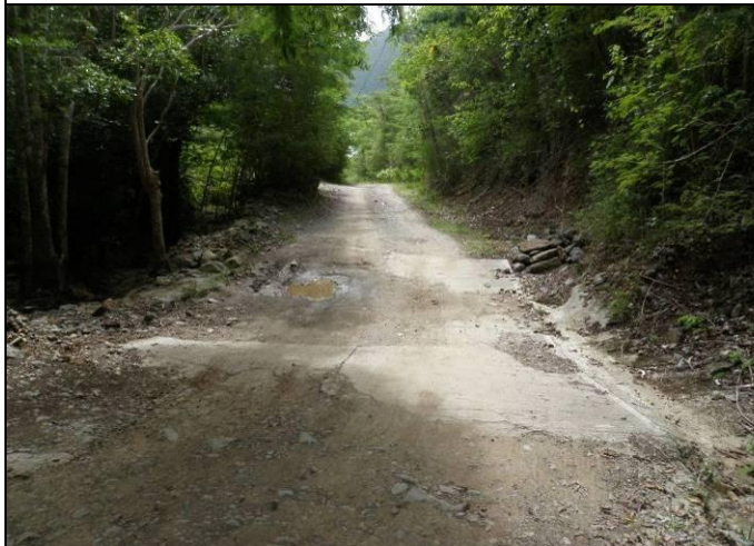
Dip intersects ditch (left side of photo) and discharges downslope (on the right). If not pitched enough or if outlet blocked by vegetation, dip can fill with sediment.
