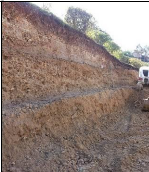
Creating benches on an almost vertical slope.
