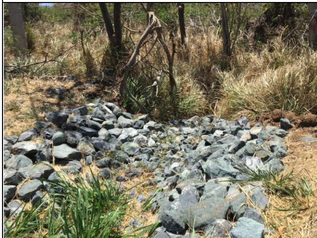
Rock aprons at outlet pipes are good if you have a level area where flow can be dissipated into a vegetated buffer.
