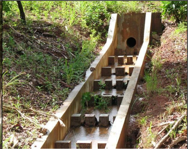
Probably overkill for short road segment outlets, but more formal energy dissipation for higher volume flows is an option.
