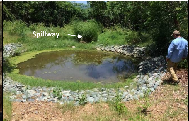
Traps can become permanent drainage control features that provide water quality treatment prior to discharge.
