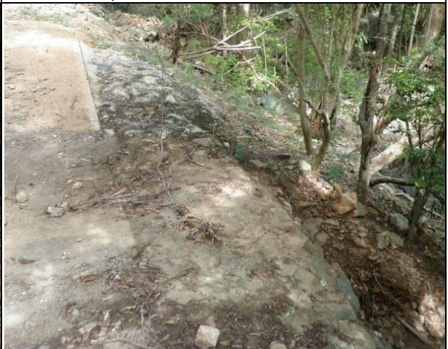
Outlet should be stabilized and include a level spreader (as shown here) or energy dissipater to slow and spread discharged flows.
