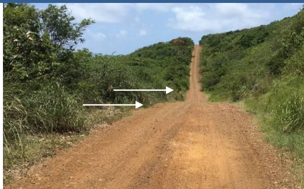
Grade Break: using subtle elevation changes to break up surface drainage areas.
