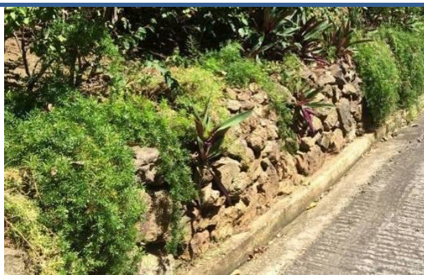
Slope Stabilization. Vegetation, stone, matting, or combination of techniques to prevent erosion of cut or fill slopes.
