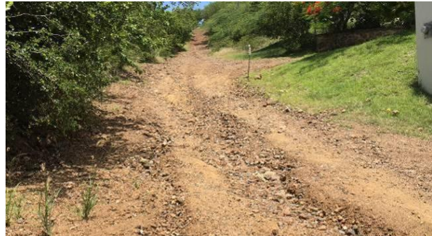
Figure 5. Common Erosion Patterns on Unpaved Road
