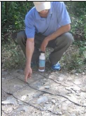
When exposed, add a thin layer of surface aggregate.
