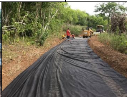
Step 2. Installation of overlapping geotextile fabric.
