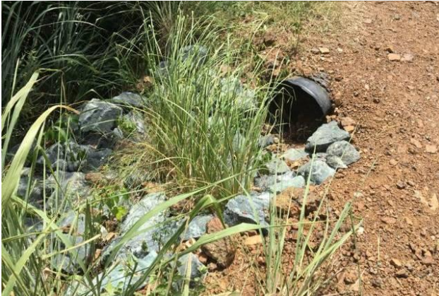
Stabilized Outfall: stone, vegetation, or other method of preventing scour at outlet structures.
