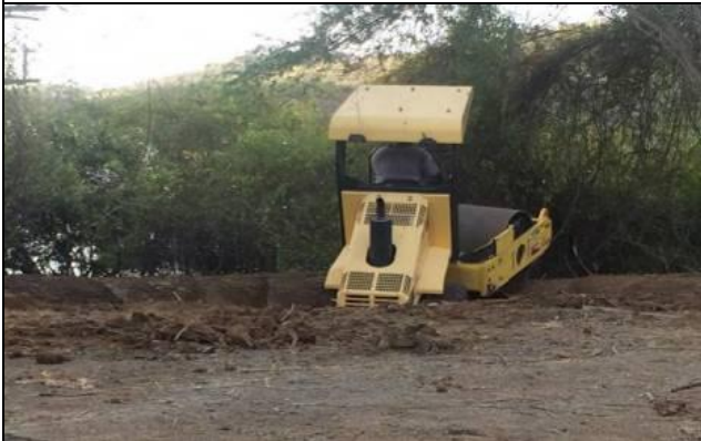
Proper compaction of dam/outlet berm with roller or hand held compactor is a critical step in construction.
