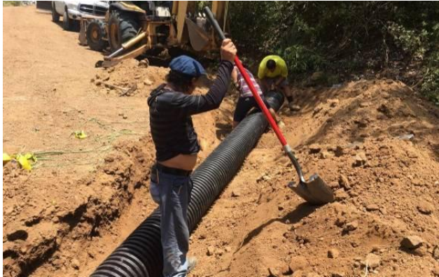
Cross-drain: piped or open top culvert that conveys concentrated flows from one side of road to other, usually from an inside ditch to the outslope.
