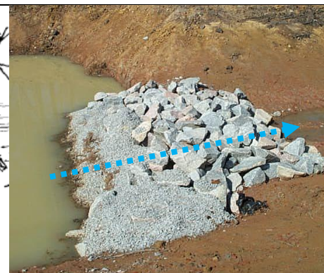
Create a filter using smaller sized rock on the inside of rock dams.
