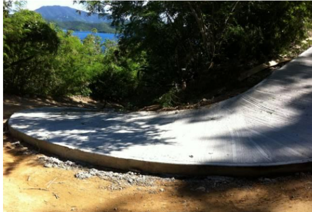
Strategic Paving: Paving sections of road that are highly susceptible to erosion, such as steep inclines and turns.
