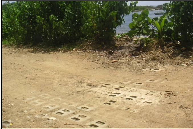
Use of concrete block dip at low point as a low cost and more "pervious" alternative to concrete.
