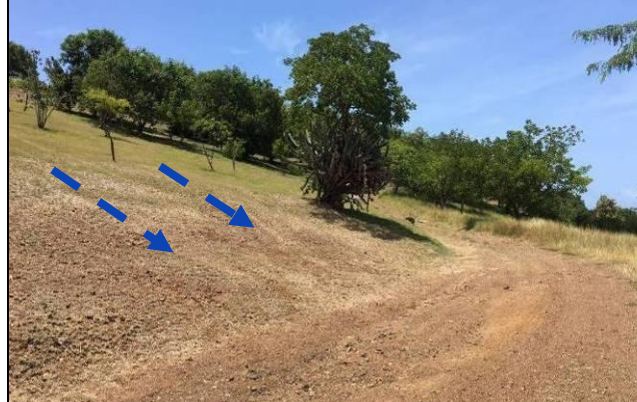
Additional flow coming from the hillside adds runoff onto the road.
