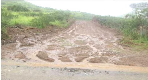
Figure 5. Common Erosion Patterns on Unpaved Road
