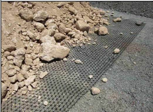
Geogrid installed between subgrade and surface layer to strengthen soil and better distribute loads.
