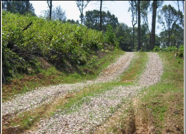
Rock reinforced broad-based dips are easily traversed by cars. Notice no ditch interception here, so concrete not necessary.
