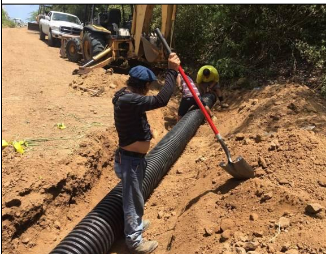
Cross-pipe installation trench should be deep enough to match ditch invert and natural ground level.
