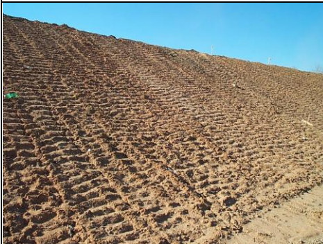
Tracking upslope to create horizontal cleat depressions across slope surface.
