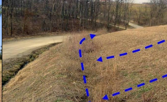
Use of an interceptor ditch would be ideal to divert runoff away from the road surface.
