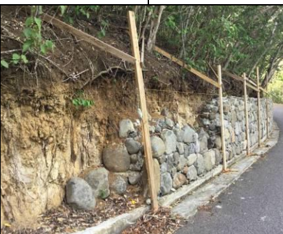
Example of a stone revetment used to stabilize road banks. Gabion baskets are also popular. Consider options that combine both rock with native vegetation.
