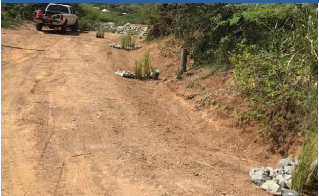
Ditch: parabolic, V-cut, or trapezoidal channel adjacent to road used to convey concentrated flows; usually has check dams and is vegetated or stone lined.
