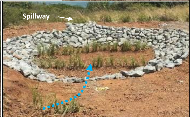
Trap design variant with rock-line side slopes and overflow spillway with vetiver grass on bottom.
