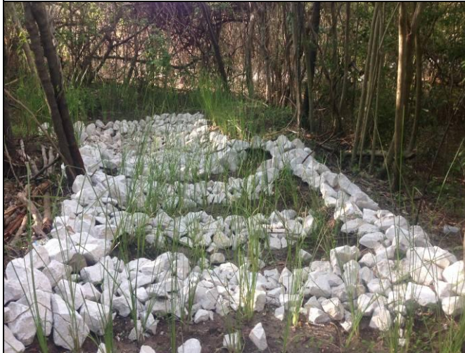
Design variant of a rock channel outlet using combination of rock and vetiver rows to dissipate flows.
