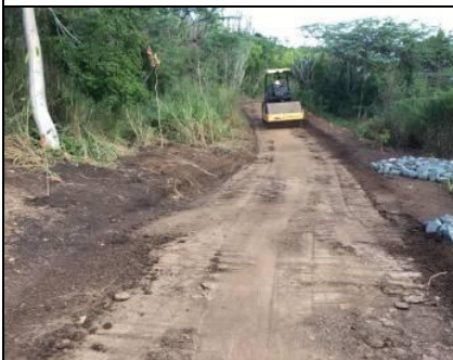
Step 1. Compaction of native subgrade.
