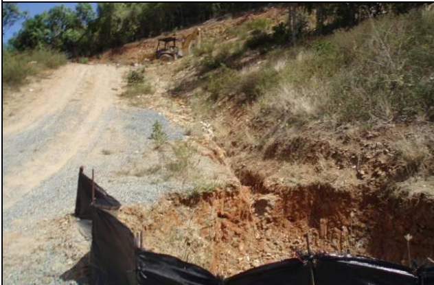
Traps built in-line with ditches can blow out with heavy rains due to lack of bypass alternatives.
