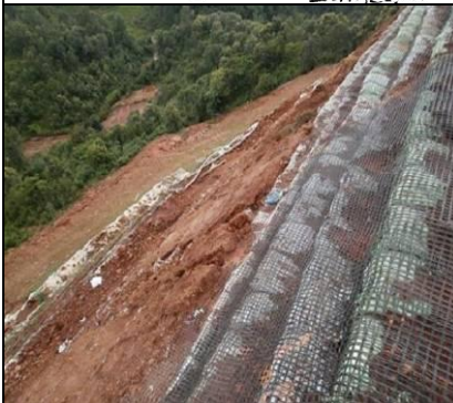
Geogrid layers stacked on a slope.
