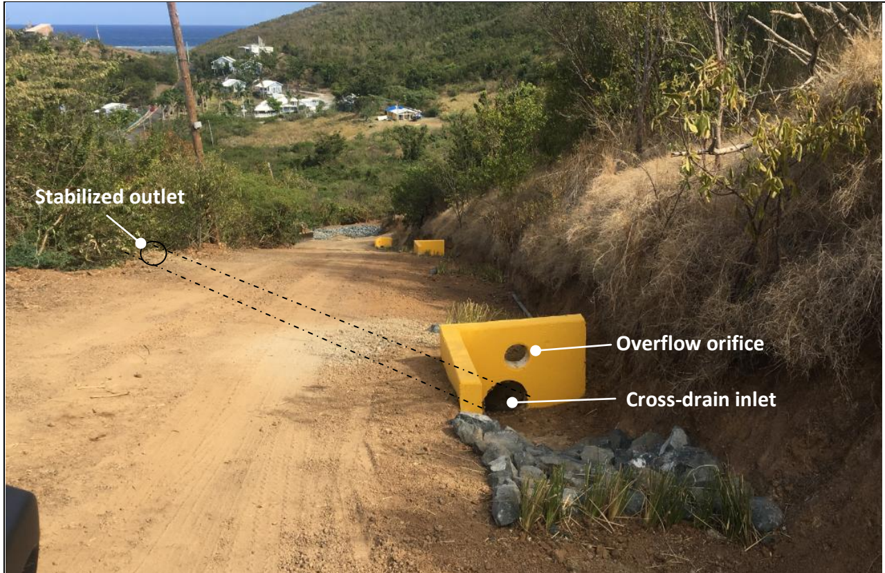
Use of headwalls for cross-drains on Culebra, Puerto Rico to increase visibility and stability around pipe inlets. The headwall helps to funnel flow into pipe. An overflow orifice is provided in case inlet becomes clogged.
