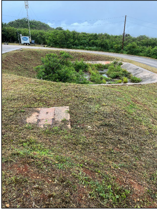
Picture 9: Concrete/earthen ponding basin near southwest quadrant of PACBAR III site
