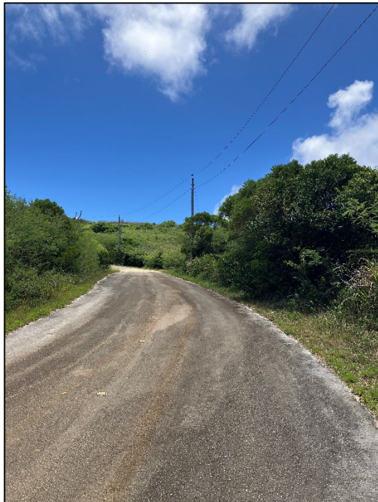
Picture 3: Existing single-phase electrical line distribution (ELD) wooden poles along Pale Arnold Road.
