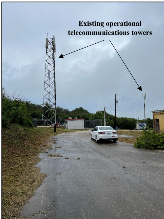
Picture 7: PACBAR III Facility Site. Existing operational telecommunications towers shown in background.
