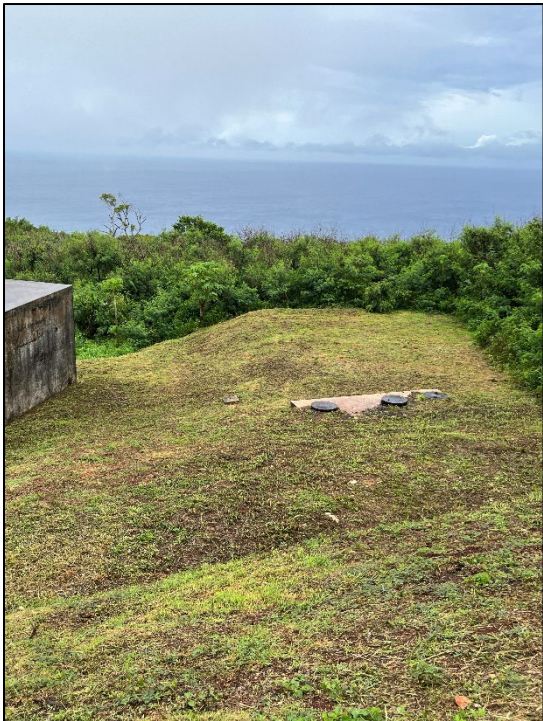
Picture 11: Likely septic tank manholes at PACBAR III site
