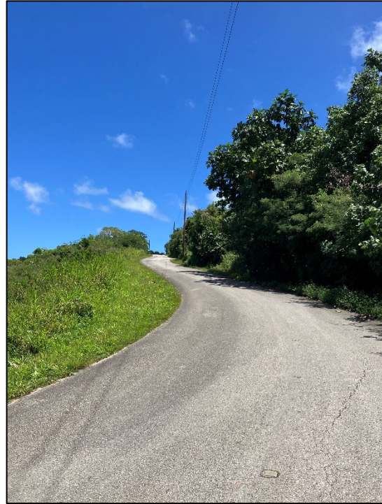
Picture 2: Existing single-phase electrical line distribution (ELD) wooden poles along Pale Arnold Road.
