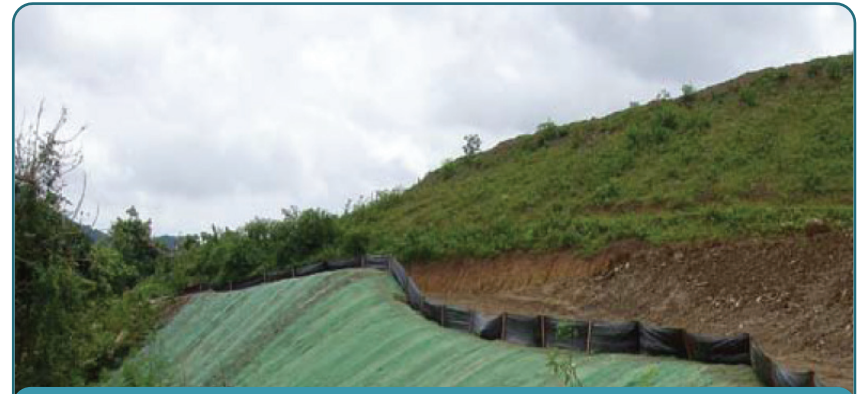
THIS: Stabilize sloped soils with fabric or erosion control blankets to hold soil in place.
