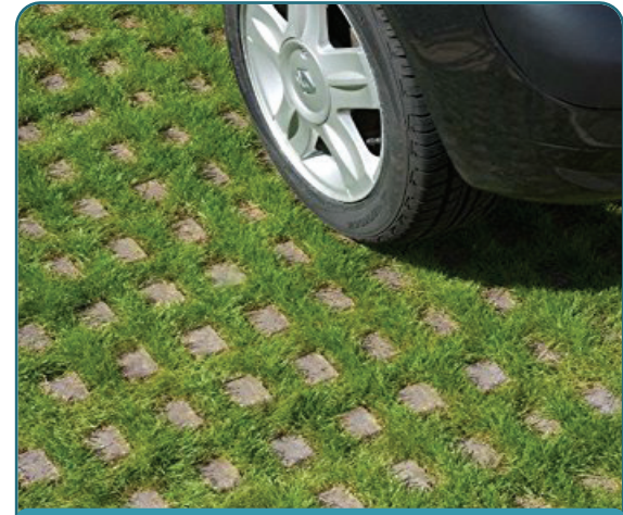
THIS: Pervious paving.
