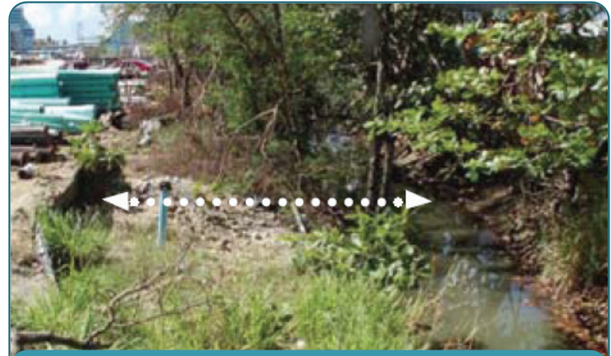
NOT THIS: The construction site is too close to the stream and lacks physical barriers to protect the stream from stormwater.
