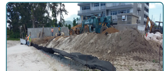
NOT THIS: Construction fence is not properly anchored.
